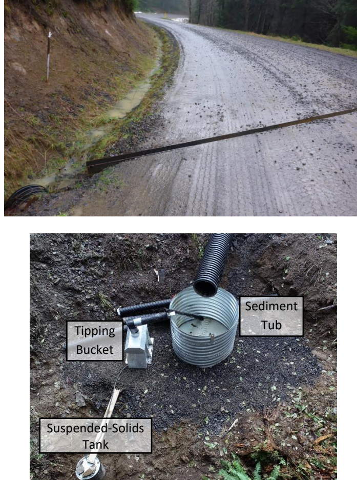
Figure 1.4 The upper image shows the road surface routing water to the ditch and the collection trough. Water and sediment then are routed through a culvert pipe to the sediment tub platform. The lower image shows the sediment tub platform with the sediment tub collecting road sediment, the tipping bucket measuring discharge, and the suspended-solids tank (SST) sampling the fine sediment that is not settled in the sediment tub.
