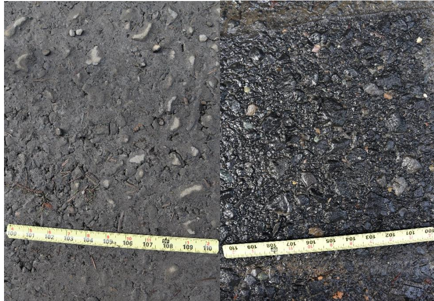
Figure 5.4 A comparison of a road surface with abundant fine sediment on the gravel on the left image. On the right is an adjoining road segment surface that was washed clean of the fine sediment to expose the gravel.
