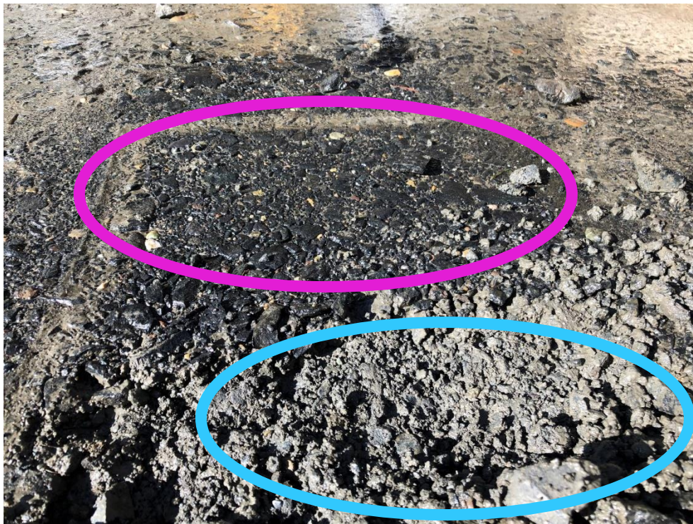
Figure 5.5 A comparison of the armoring of the surface (circled in pink) in contrast to the abundant fine material in the subsurface (circled in blue).
