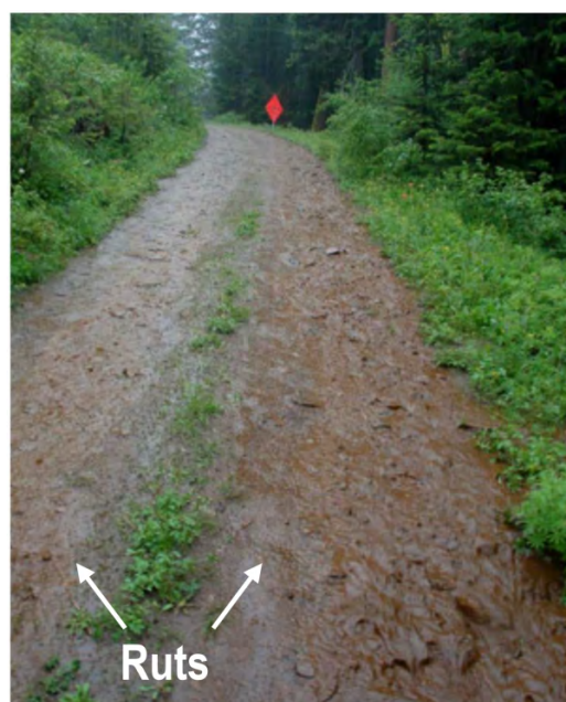
Fig. 6. Image of an extremely rutted road that receives little traffic.
