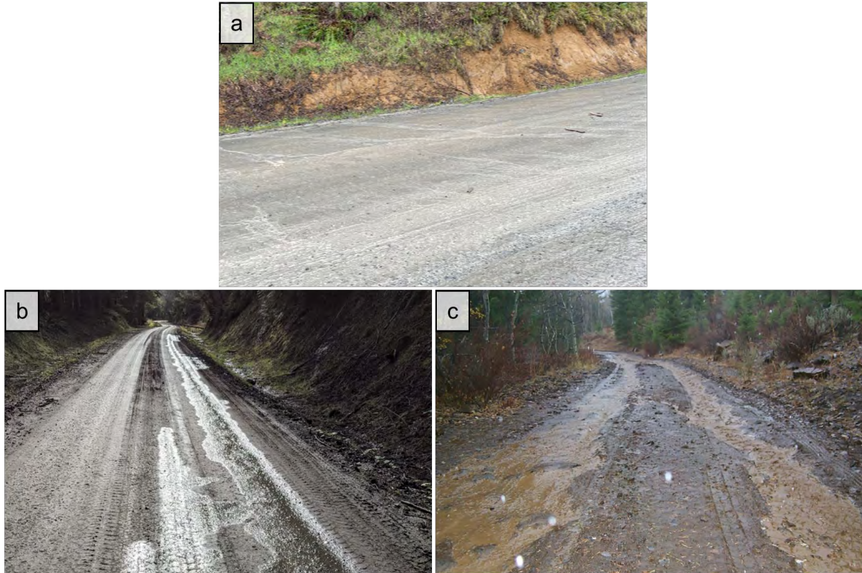
Figure 2. Example photos of (a) an un-rutted road with flow heading to the ditch line from the center of the road; (b) water traveling down-road in a wheel rut instead of being directed to the roadside ditch; and (c) a heavily rutted road with channelized, sediment-laden flow heading down-road. The road widths seen in each of these photos are approximately 5 meters.
