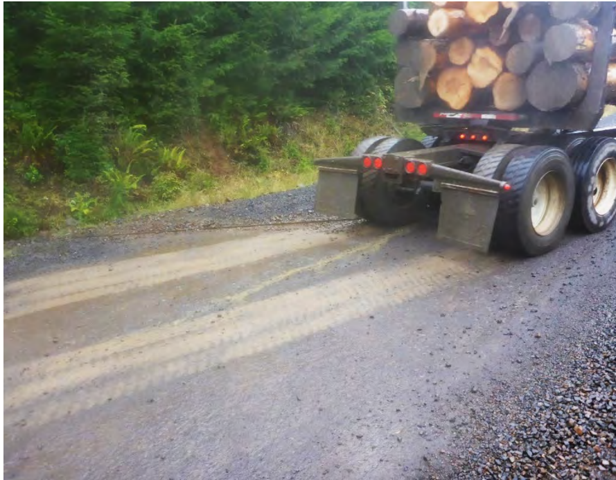
Figure 6.1 New fine sediment pumped from the roadbed by the passage of a loaded log truck.
