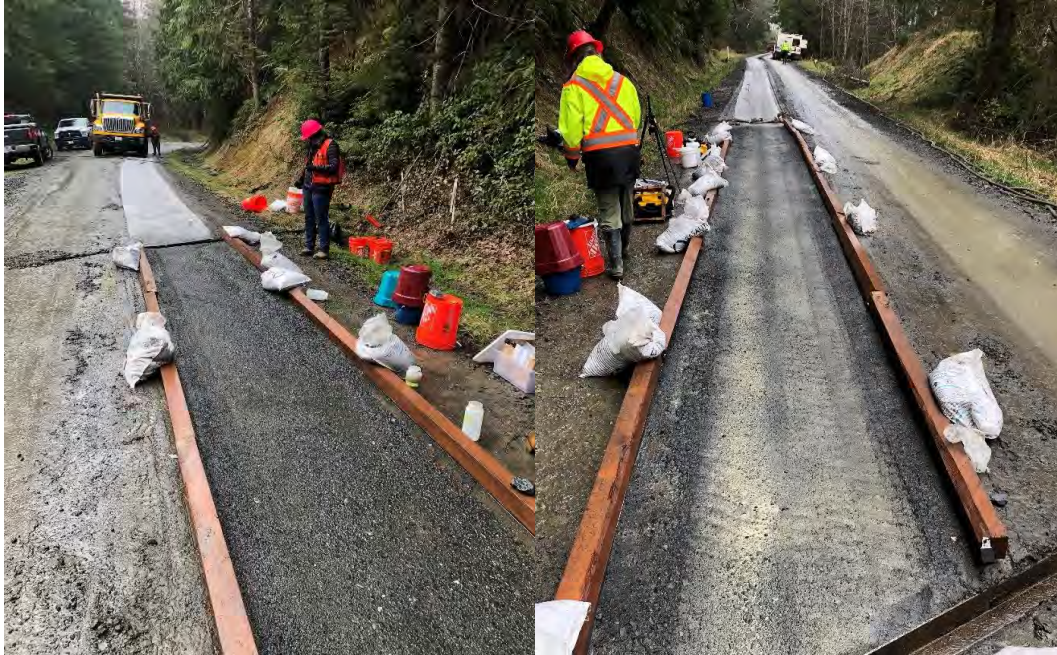
Figure 6.2 Surface and the photo on the right shows the surface after 6 truck passes.
