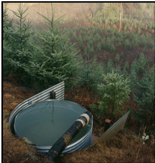
Figure 2: A sediment trap installed below a road segment.
