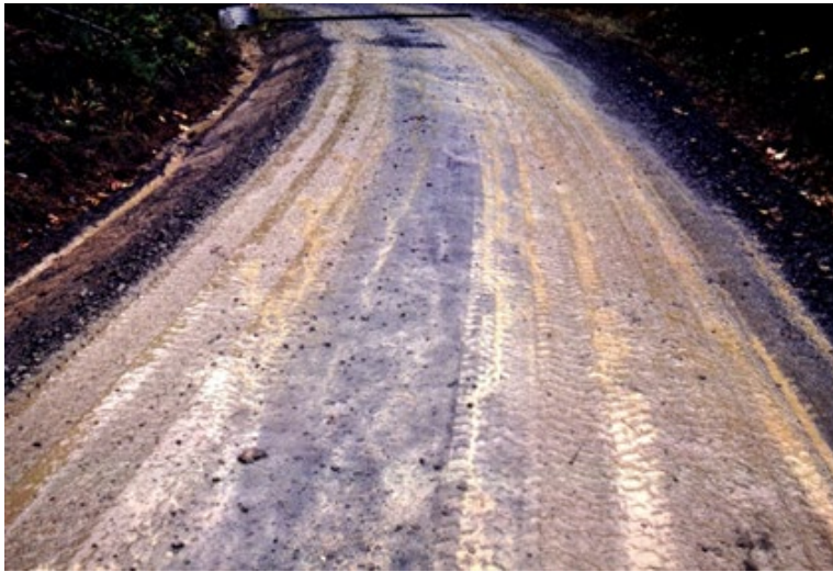
Figure 8. An example of a wet forest road surface after trucks have passed. The sediment in the upraised patterns are fine sediments that were pressed into tire sipes and would be easily transported if it were raining.
