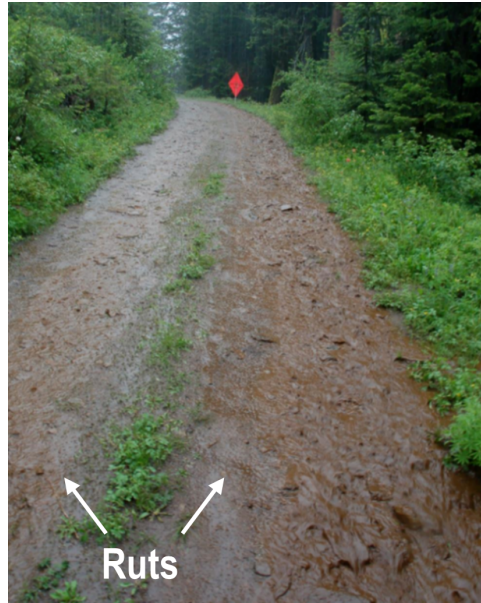
Figure 2.6: Image of an extremely rutted road that receives little traffic.
