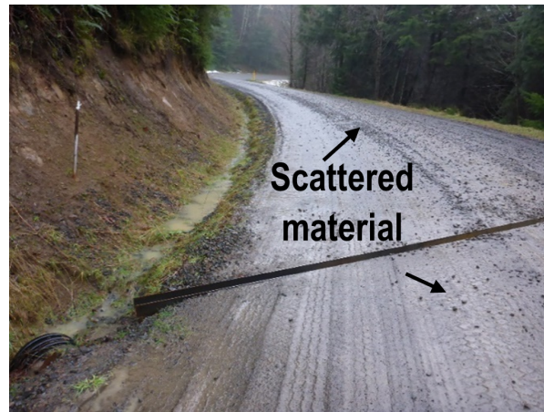
Figure 2.4: Image of a forest road with evidence of scattering.
