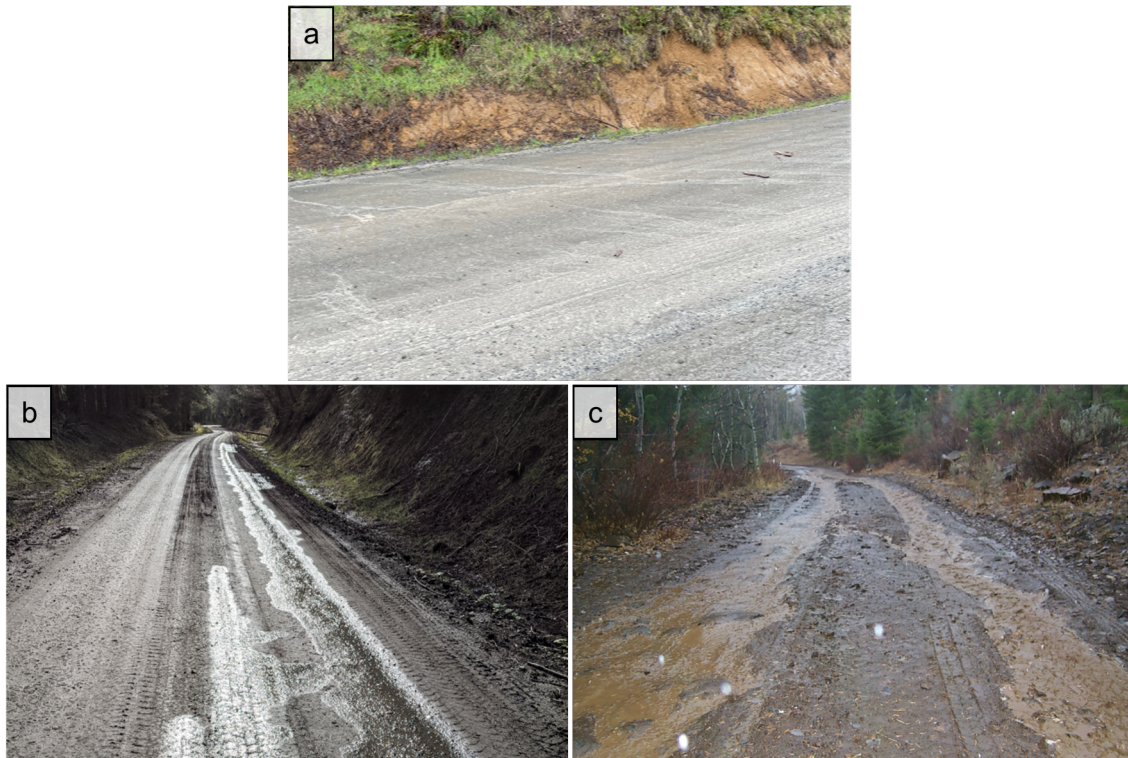
Figure 4.2: Example photos of (a) an un-rutted road with flow heading to the ditch line from the center of the road; (b) water traveling down-road in a wheel rut instead of being directed to the roadside ditch; and (c) a heavily rutted road with channelized, sediment-laden flow heading down-road.
